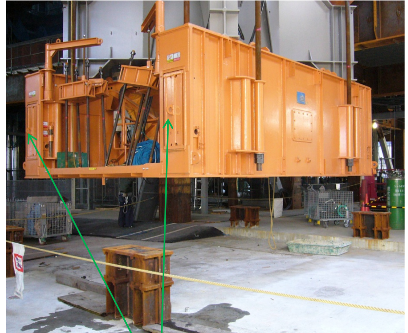
retracted outriggers during climbing
