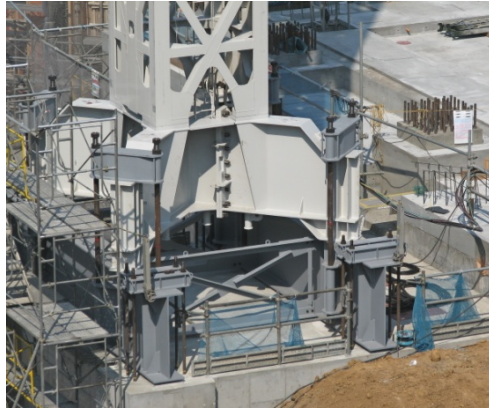
external crane base
