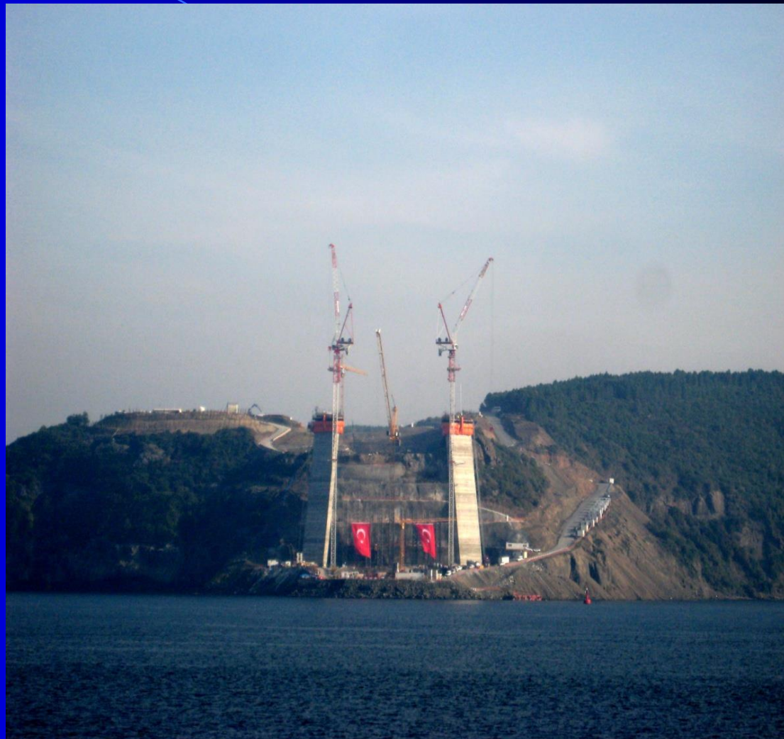
THIRD BOSPHORUS BRIDGE – TURKEY
