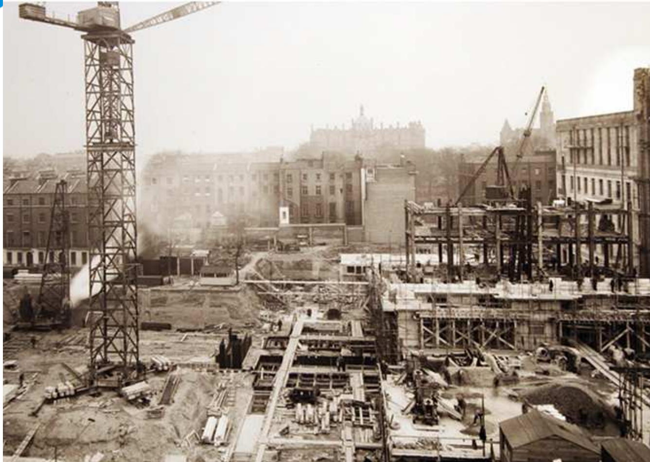
Senate House construction site, London University, c1935
