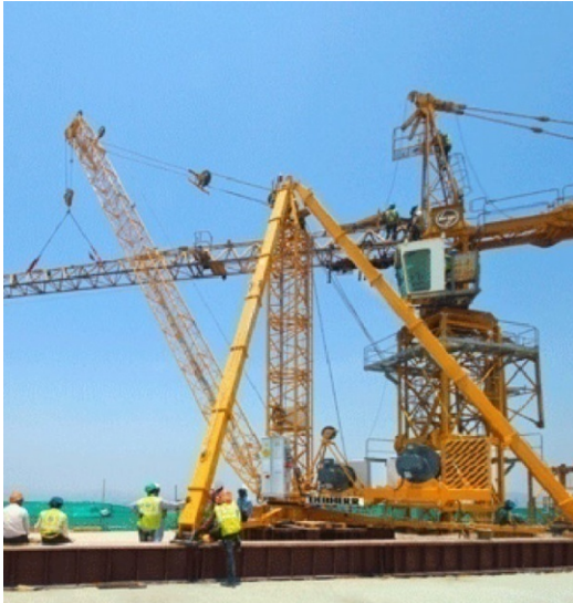
derrick configuration with outrigger extension and stifflegs
