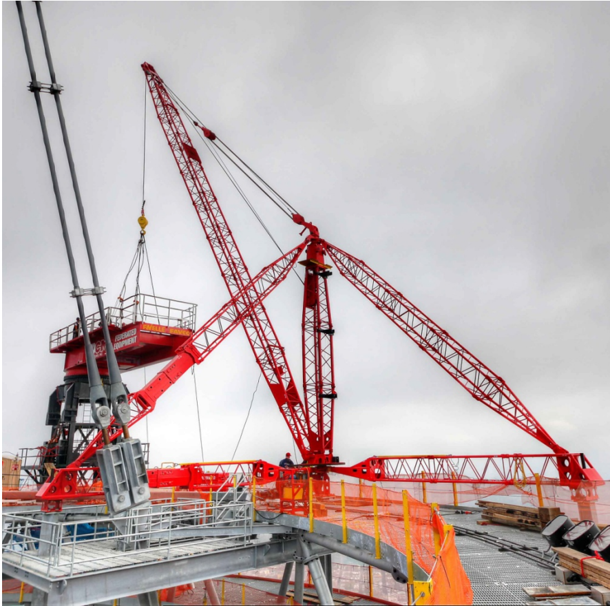
Timberland ASD11-110 adjustable stiffleg derrick
