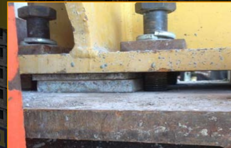
Metal- concrete match
