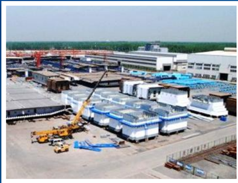
Prefabricated Modular Construction
