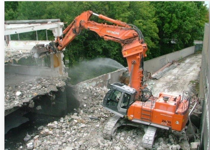
Demolition two-piece-boom (back side)
