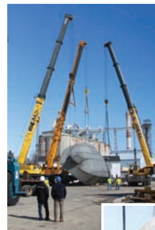
The three cranes picked up and rolled the ship's hull.
