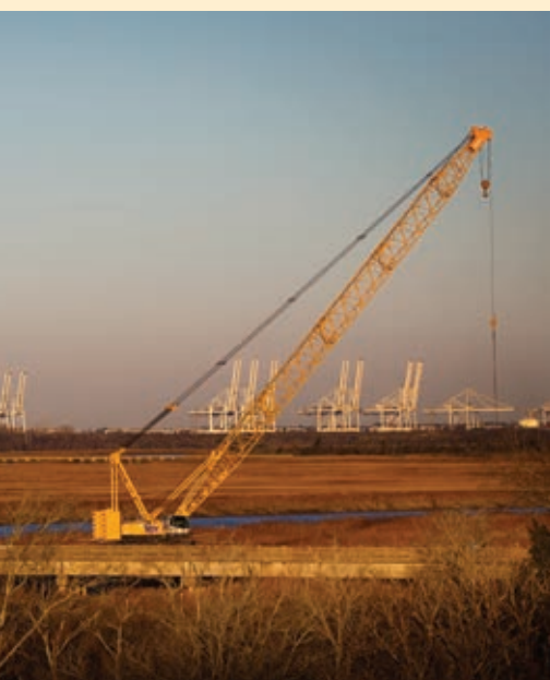
PHOTO: Dozier Crane
