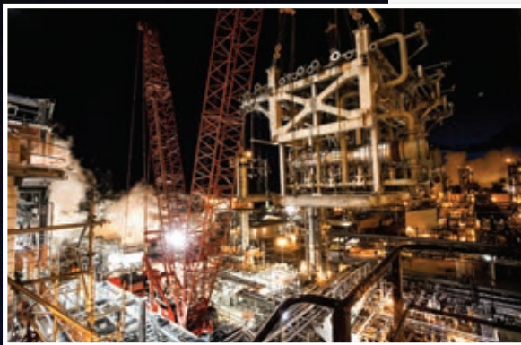
Due to the small window of time allowed for the project, work was performed around the clock. One of the modules ended up flying at night.
