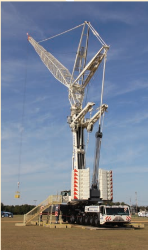
PHOTO: Deep South Crane & Rigging
