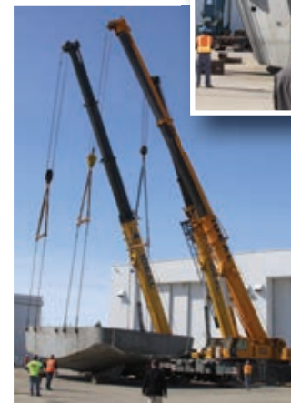
The three cranes picked up and rolled the ship's hull.
