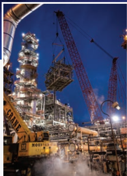
A Grove RT530E was used as an assist crane on the project.
