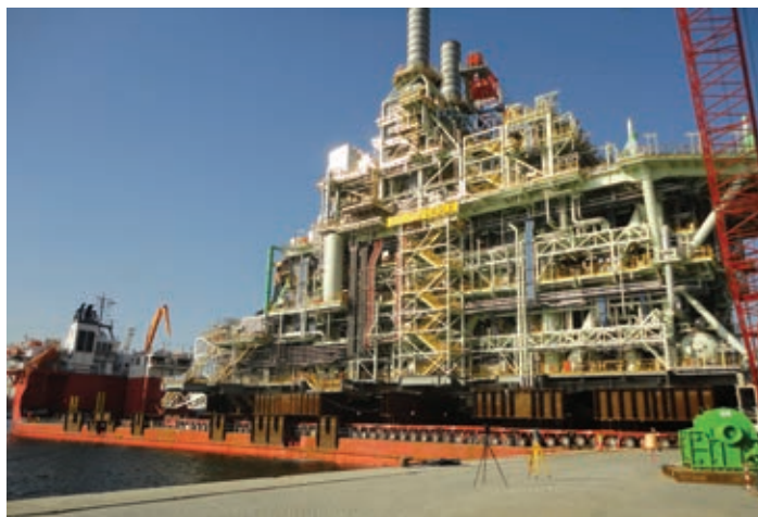
ALE used 512 axles of SPMT to move an offshore platform.
