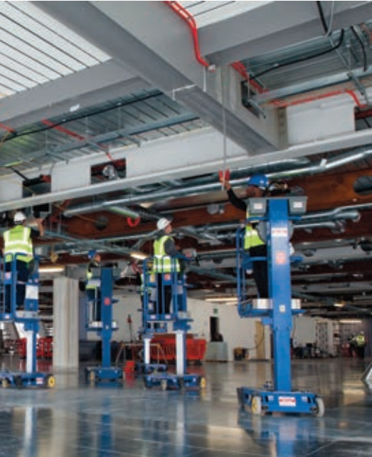
Pecolifts in use at the UK£50 million fit-out of the News Corporation building (Baby Shard), Southwark, London, UK. Main contractor is ISG.
