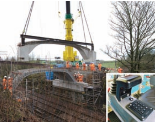
Contractor BAM Nuttall has fitted Kosran's Safety Access Control system (SAC) on its crawler crane fleet, ensuring that only authorised workers can operate the machines.
