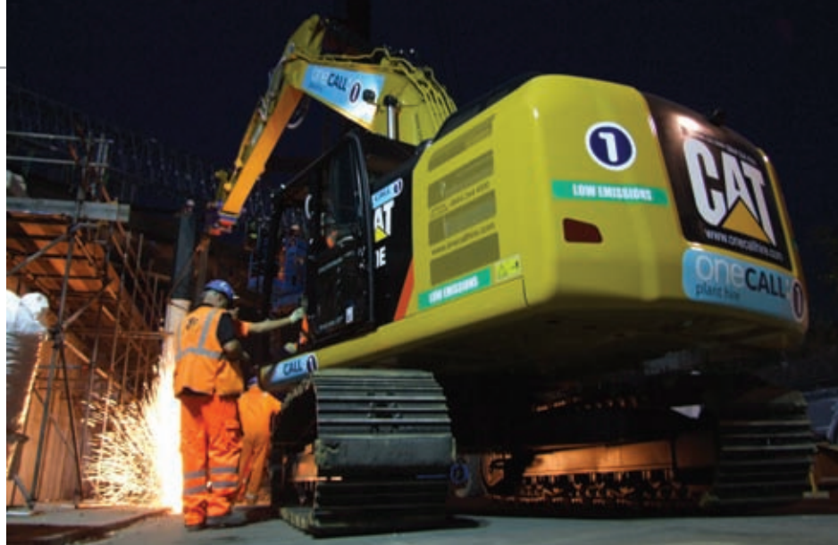
In the UK, One call Hire is making a point of buying Stage IIIB excavators for its hire fleet.
