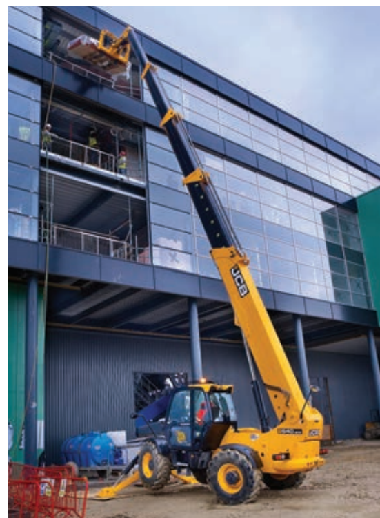
JCB's 540-200 lifts construction materials into place
