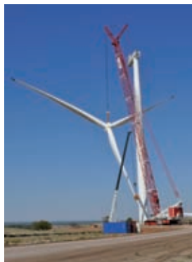
CC 2800 at a windmill construction
