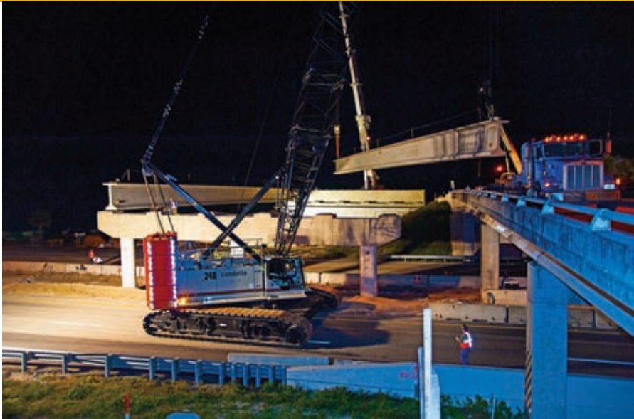
Condotte America Inc. used a 200-ton Link-Belt 248 HSL to complete beam placement for a bridge project on the Florida Turnpike. The crane was rigged with 165 feet of main boom and 172,000 pounds of counterweight to place 12 I-beams from 104 to 140 feet in length.
