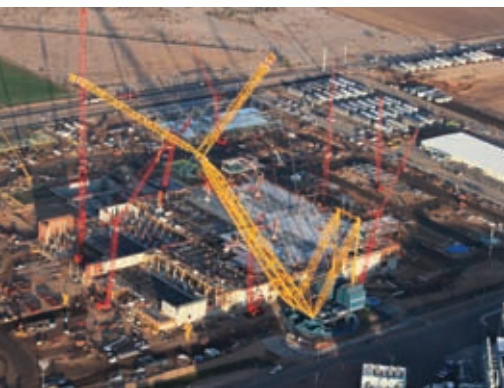
After working at its inaugural job at a construction jobsite in Arizona, the Sarens SGC-120 went to work in China.
