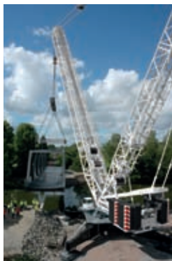
PC 6800 at a bridge construction
