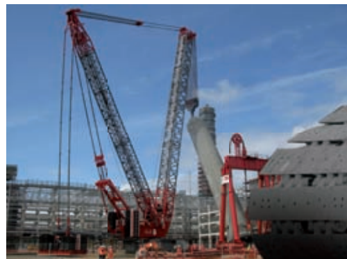
CC 8800 at an oil refinery construction
