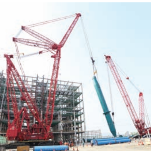
The first Manitowoc Model 31000, with a capacity of 2,535 tons, works at its first job at Posco E&C plant in Gwangyang, South Korea.
