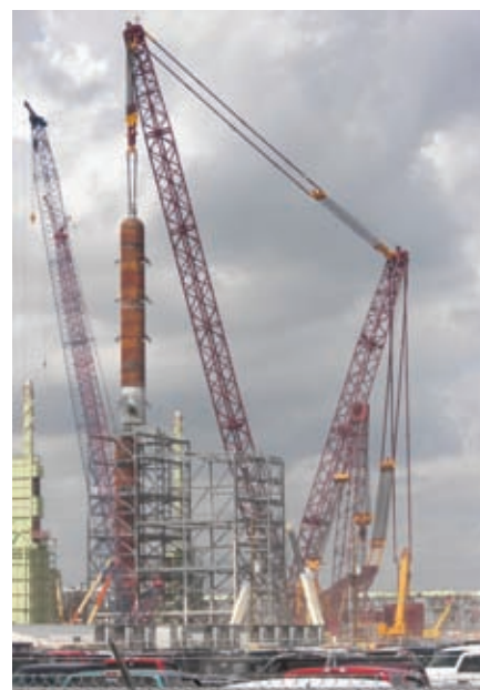
Deep South's VersaCrane TC-36000/1 has a capacity of 2,500 tons.
