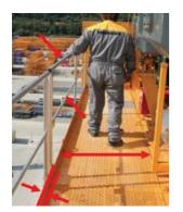
5.4 Toe-boards, handrails and access
