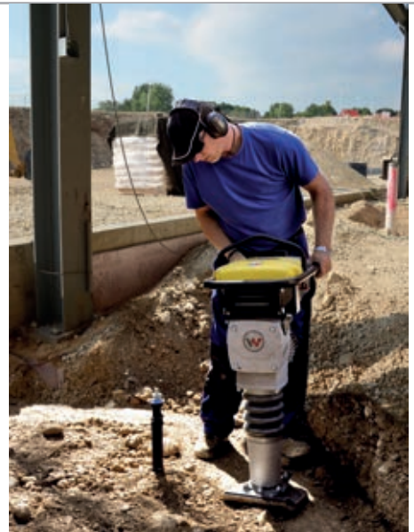
Wacker Neuson's new battery-powered AS 50 rammer
