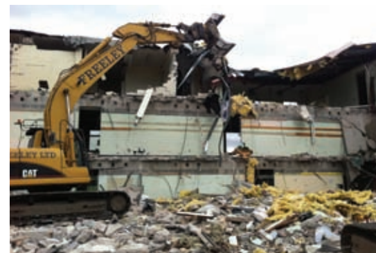
UK contractor J Freeley has completed its sixth school demolition in two years, the latest being the Stamford Community High School
