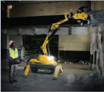
South African contractor Draco Demolition CC has invested in a Brokk 100 with a CC 320 crusher and SB 152 breaker
