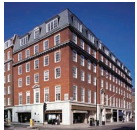
The structure was a seven storey building (including a basement level)
