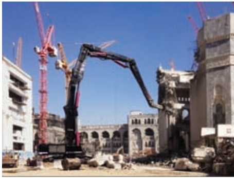
Three Rusch RS4500s are working on a mosque demolition in Mecca, Saudi Arabia – the machines were supplied in November despite Rusch Special Products entering insolvency earlier in the year (courtesy of Hélène de Bruijn Fotografie, Netherlands)
