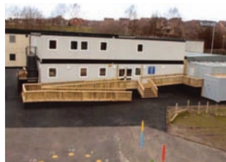
Two Storey Modular Building
