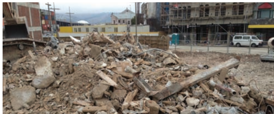
Although a 'dirty' demolition, much of the resulting 20,000 tonnes of debris was processed for recycling
