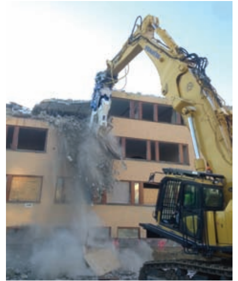
Rivners' new MK 70 from Trevi Benne at work on the old HQ building of AB Atomenergi, Nutek House
