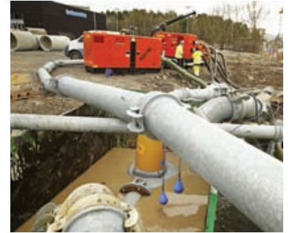
Xylem had to design a temporary, customised bypass solution
