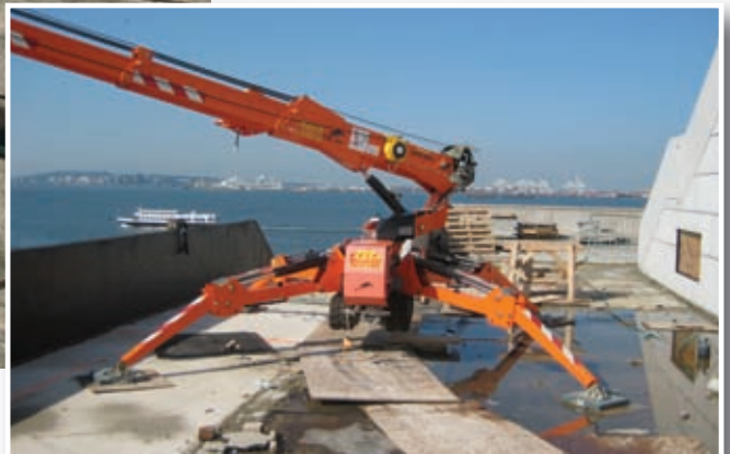
Phillipsburg Marble rented a Jekko SPD360 from Area Rentals in Hillside, NJ to perform the upgrade work on the pedestal of the statue. The project included removal and reinstallation of more than 450 granite pavers and stone wall panels.
