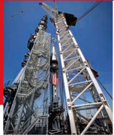
The final spire section was lifted to the roof of the building on May 2 and was erected to its final height on May 10.
