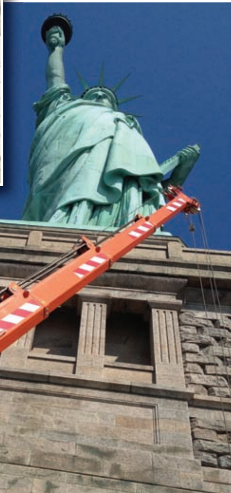
Phillipsburg Marble rented a Jekko SPD360 from Area Rentals in Hillside, NJ to perform the upgrade work on the pedestal of the statue. The project included removal and reinstallation of more than 450 granite pavers and stone wall panels.
